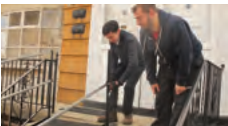
Volunteers installing a new wheelchair ramp
